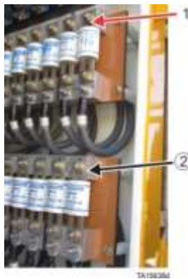
1) Positive bus bar, 2) Negative bus bar
